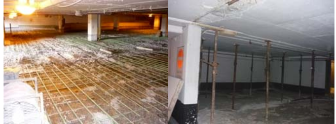
P7 Rebar & Concrete Replacement
